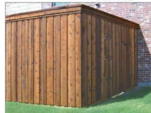
8" TALL CEDAR BOARD ON BOARD, WITH GALVANIZED STEEL POSTS AT 6" O.C. SET 4" IN GROUND IN 4" DIAMETER CONCRETE FOOTING
