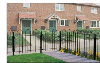
06 Patio Fence No Scale 42 INCH HIGH BLACK PAINTED WROUGHT IRON PATIO ENCLOSURE
